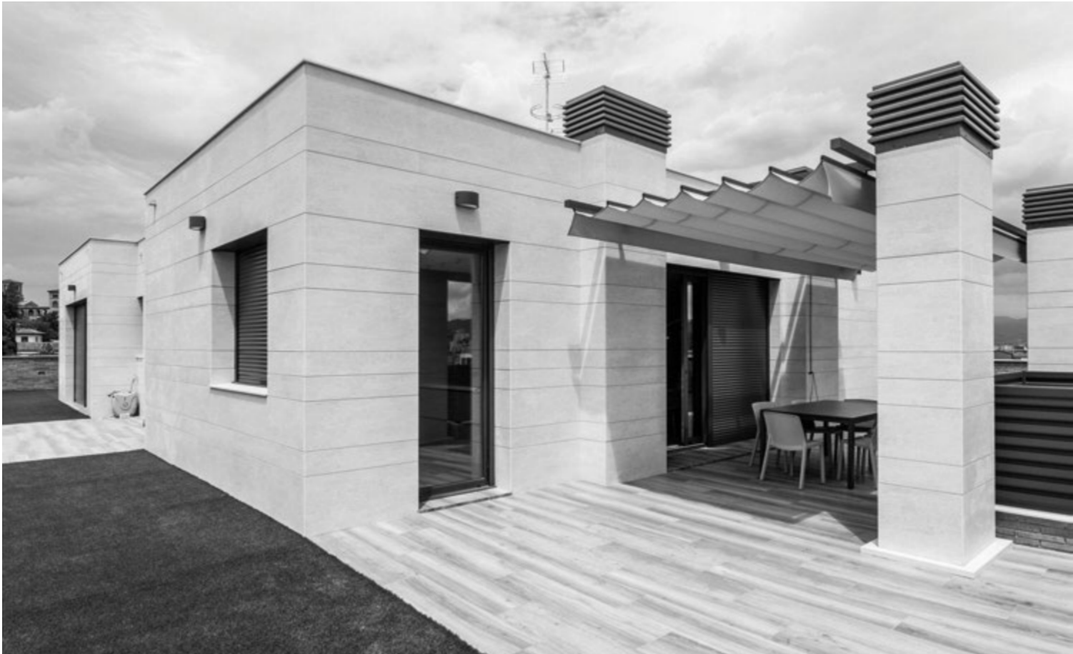
Moles Building, Girona, Spain.
