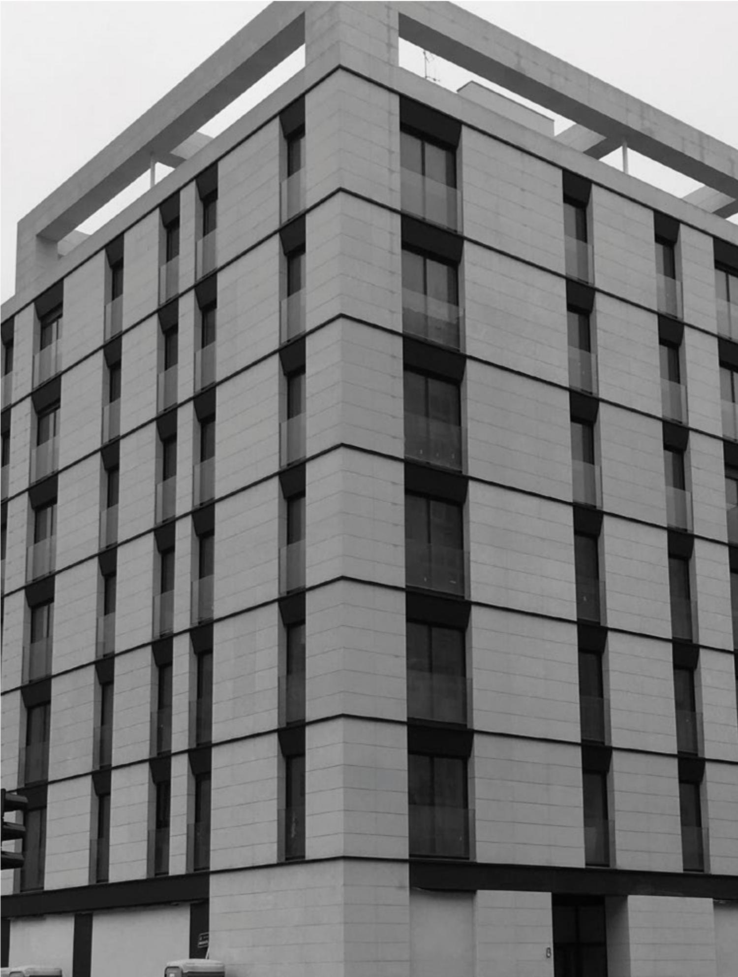
Tabacalera apartment building, A Coruña, Spain
